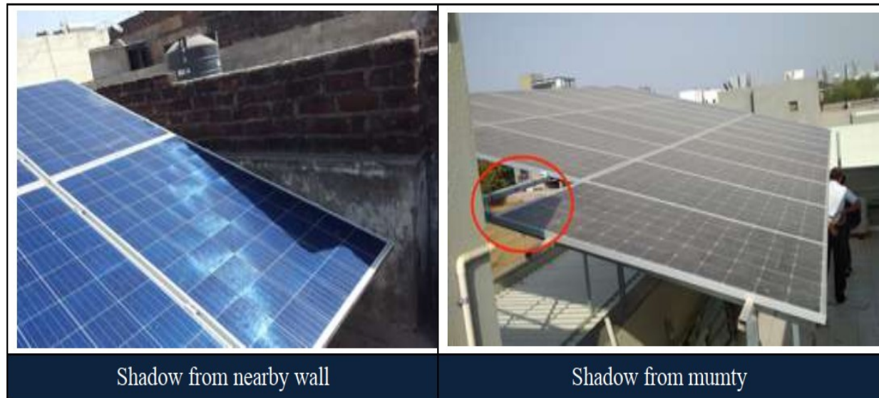
Fig.2.13: A Solar Panel Shadow Effect
